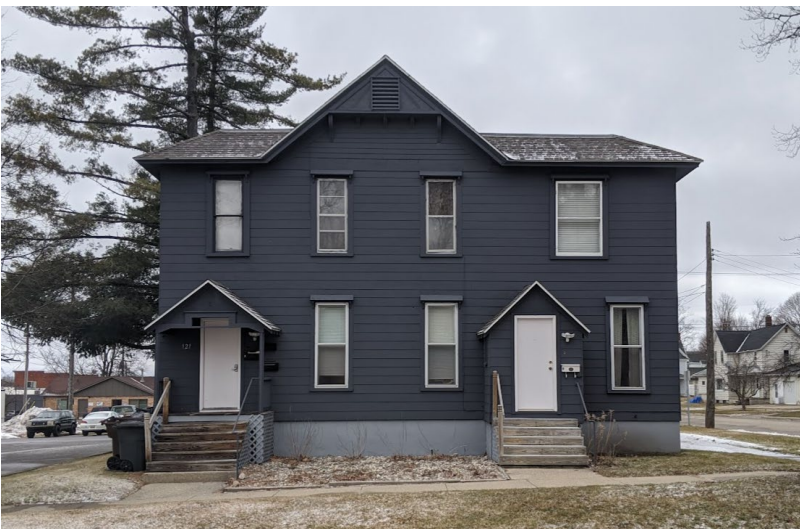
4-unit residential apartments to the North
