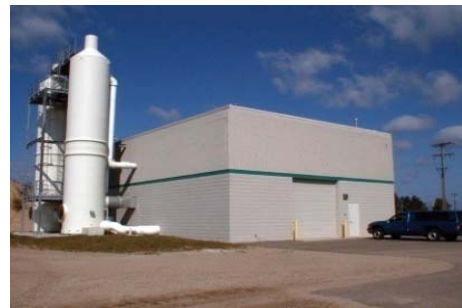
LDFA Water Treatment Facility
