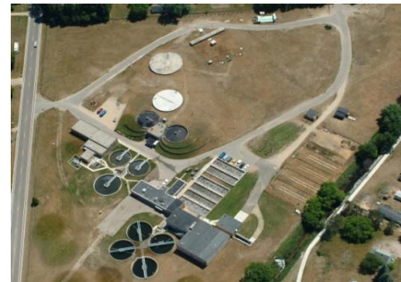
Wastewater Treatment Facility
