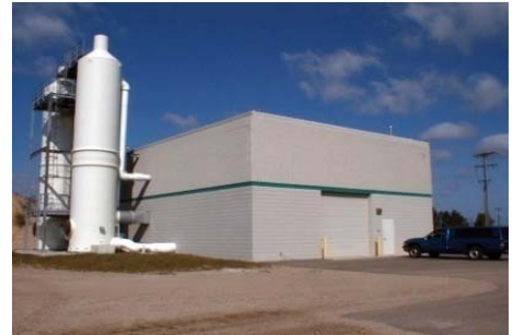
LDFA Water Treatment Facility
