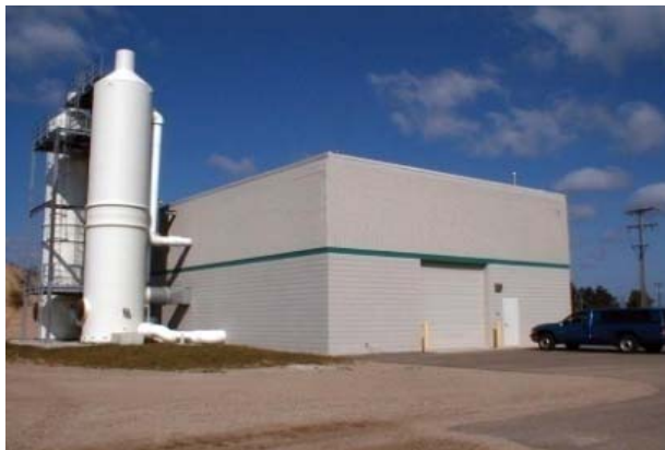
LDFA Water Treatment Facility
