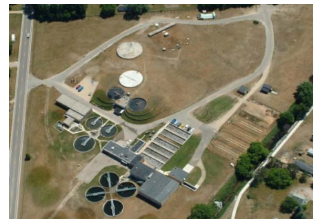
Wastewater Treatment Facility
