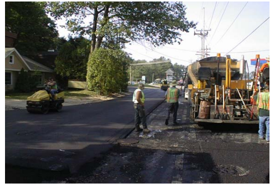
Leisure Road after reconstruction
