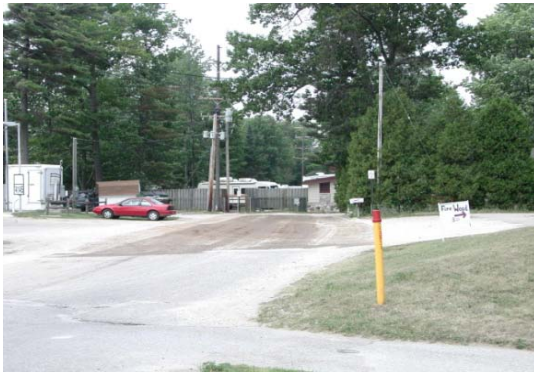
Leisure Road before reconstruction
