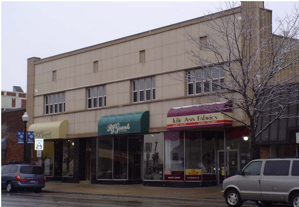
The H.L. Green Building
