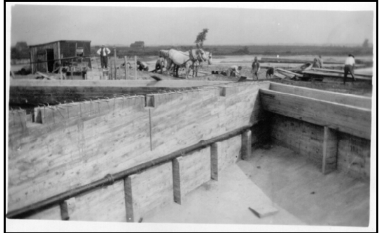
September, 1923 construction of original facilities. (Looking north at what are now CASA fields)
