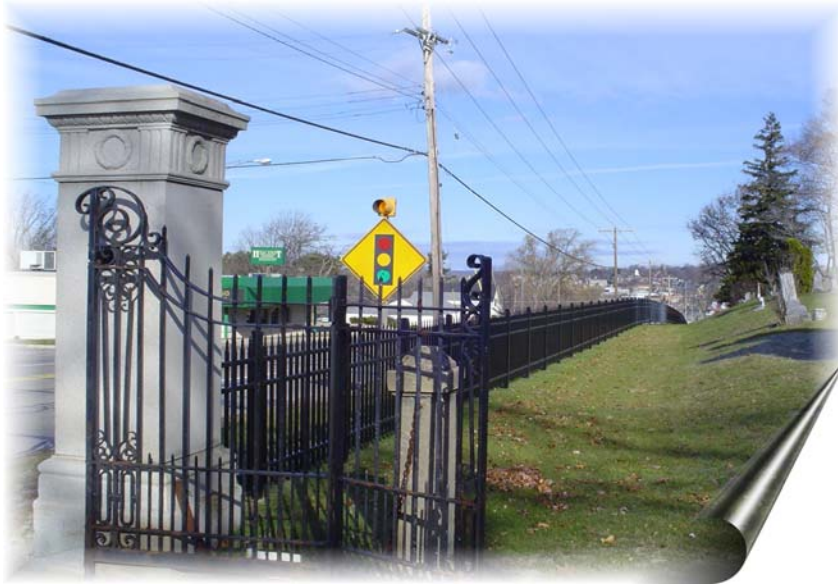
New fencing project on US-131 entrance
