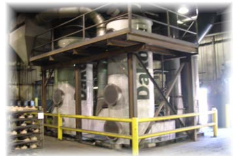
Hazardous chemicals at local manufacture are monitored
