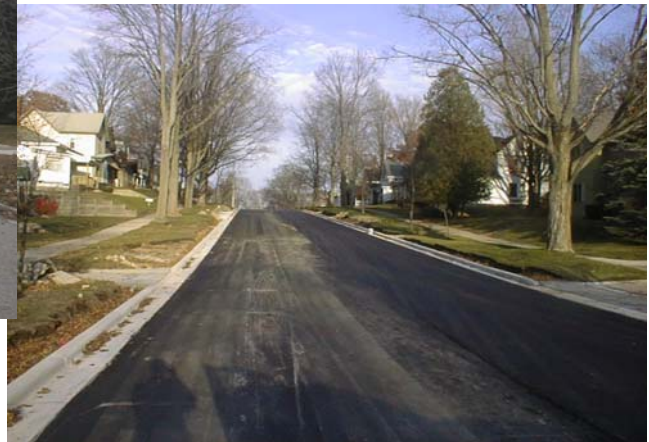
Stimson Street after construction
