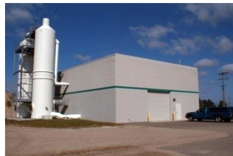
LDFA Water Treatment Facility
