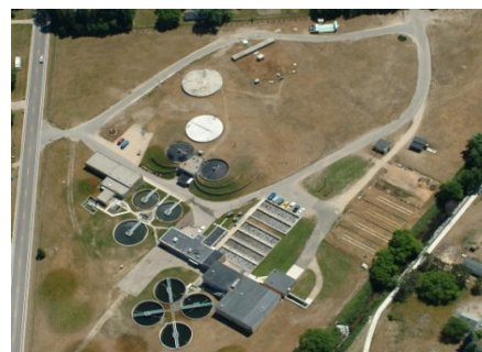
Wastewater Treatment Facility
