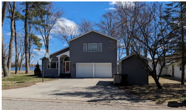
Photo of neighboring home (116 Shore Lane) with permitted storage building in the road front yard (treated as a rear yard for the placement of accessory structures).
