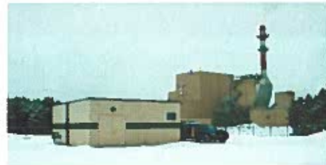
LDFA well house (foreground) with Cadillac Renewable Energy in background
