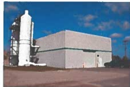
LDFA Water Treatment Facility
