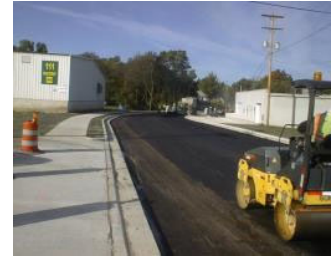
Construction activities are a big part of the long-term capital planning process.
