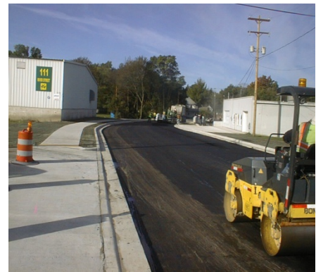
Construction activities are a big part of the long-term capital planning process.
