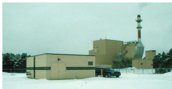
LDFA well house (foreground) with Cadillac Renewable Energy in background
