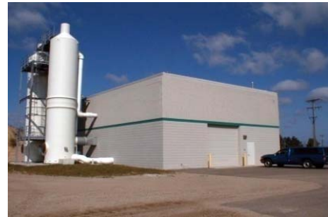
LDFA Water Treatment Facility
