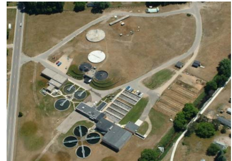
Wastewater Treatment Facility
