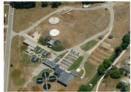
Wastewater Treatment Facility
