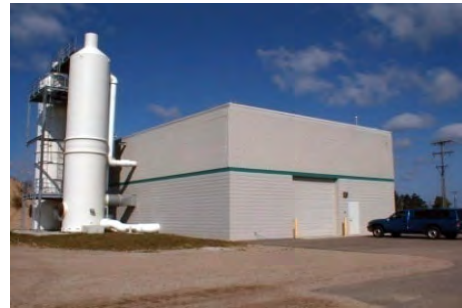
LDFA Water Treatment Facility
