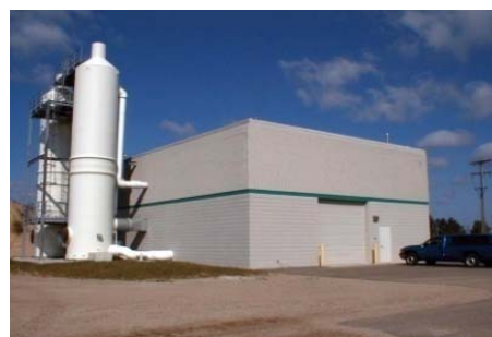
LDFA Water Treatment Facility
