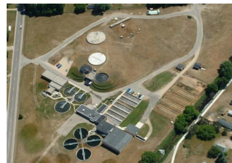
Wastewater Treatment Facility
