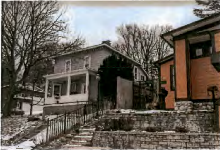
Duplex unit to the East
