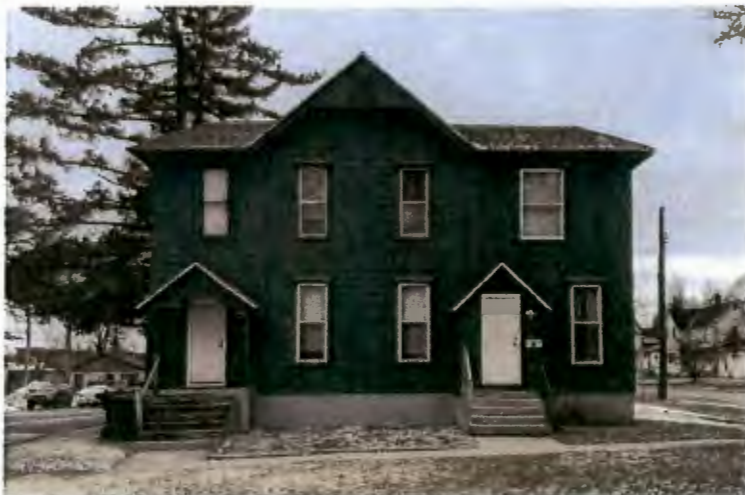
4-unit residential apartments to the North
